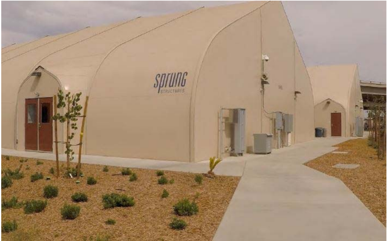
Fresno Rescue Mission – Sprung Structures
